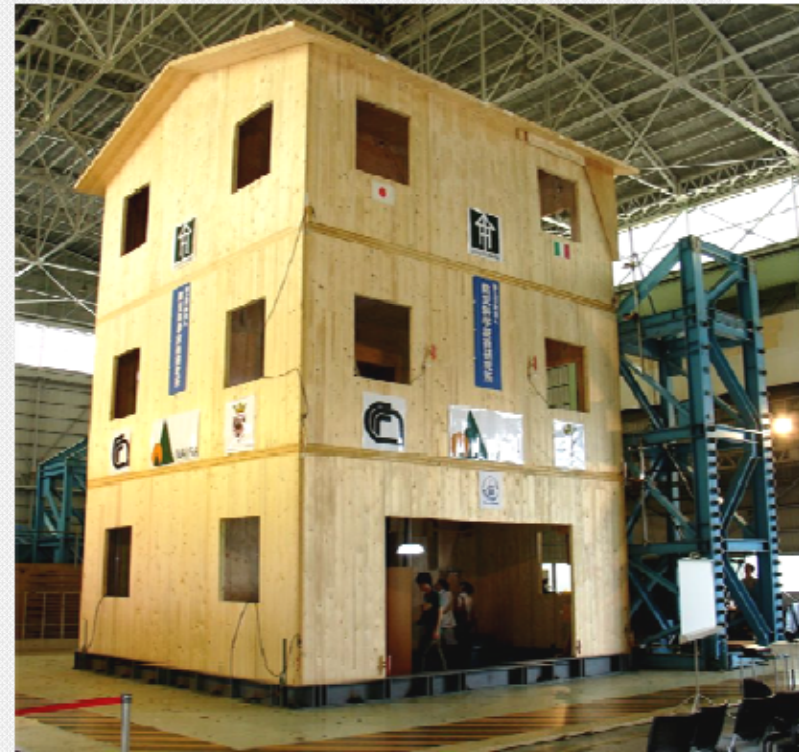
Shaking Table Test on a full- scale 7mx7mx10m of height 3 storeys XLam building
