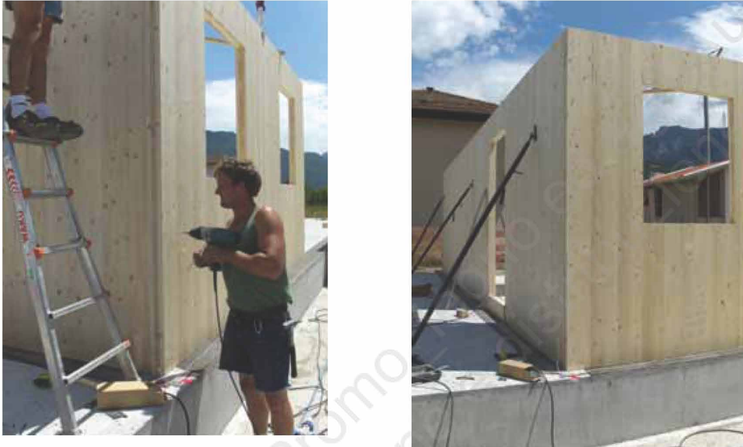
Figura 21 Collegamento parete – parete (courtesy of STP srl)
